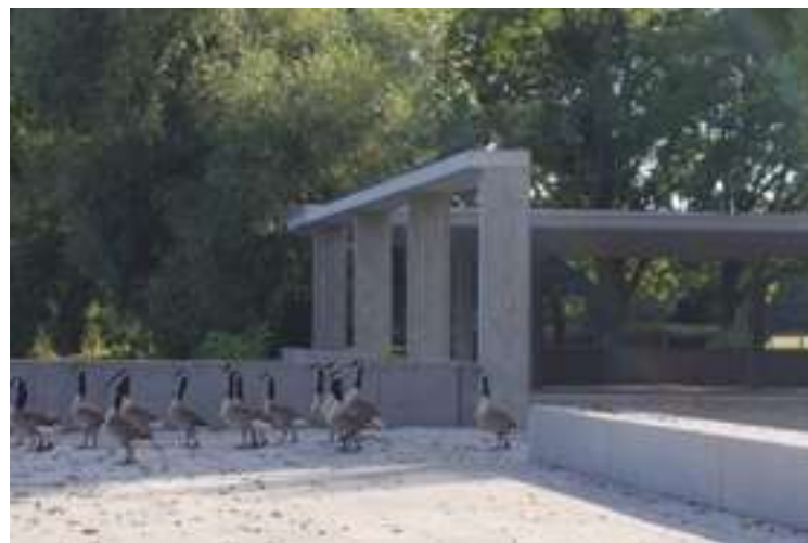
Fig. 18 Work in progress at the Cetto-Pavillon, July 2019. Photo: Suleman Anaya.
