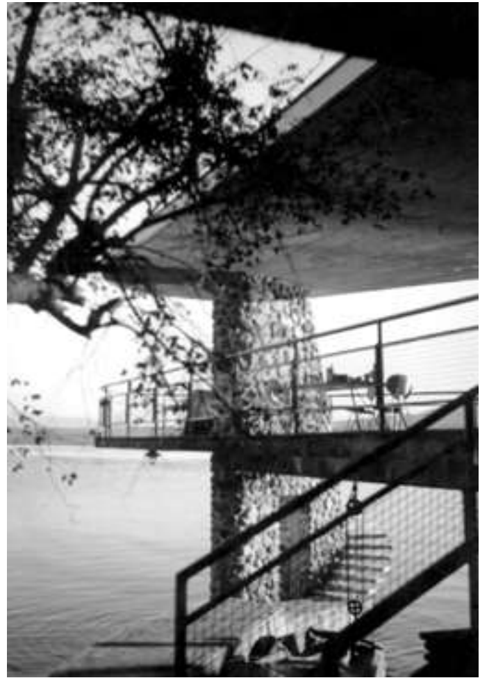
Fig. 32 Access to the terrace, Quintana House in Tequesquitengo, 1948. Photo: Max Cetto.
